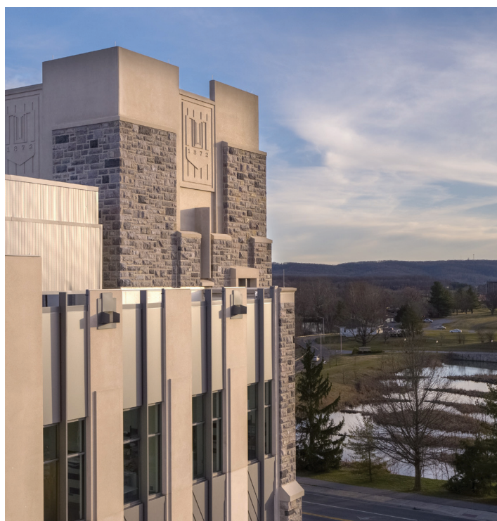
A view of the classroom building near the construction site of the Data and Decision Sciences building, the first part of the new Global Business and Analytics Complex designed to provide collaboration space to address some of the world's significant data challenges.
