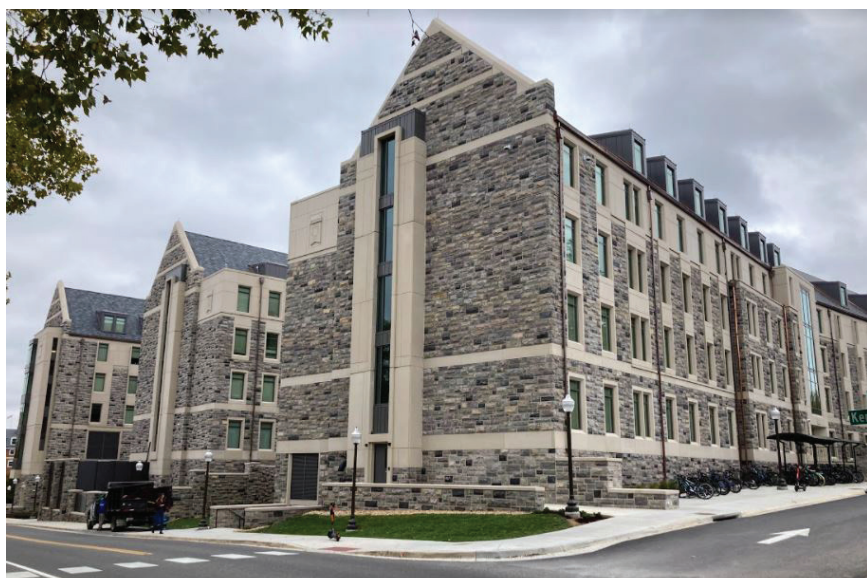
Anchoring the initial development of the Creativity and Innovation District is a 232,000 gross-square-foot residence hall, which opened in August 2021. It offers housing for approximately 600 students and various academic, social, research, and collaboration spaces.
