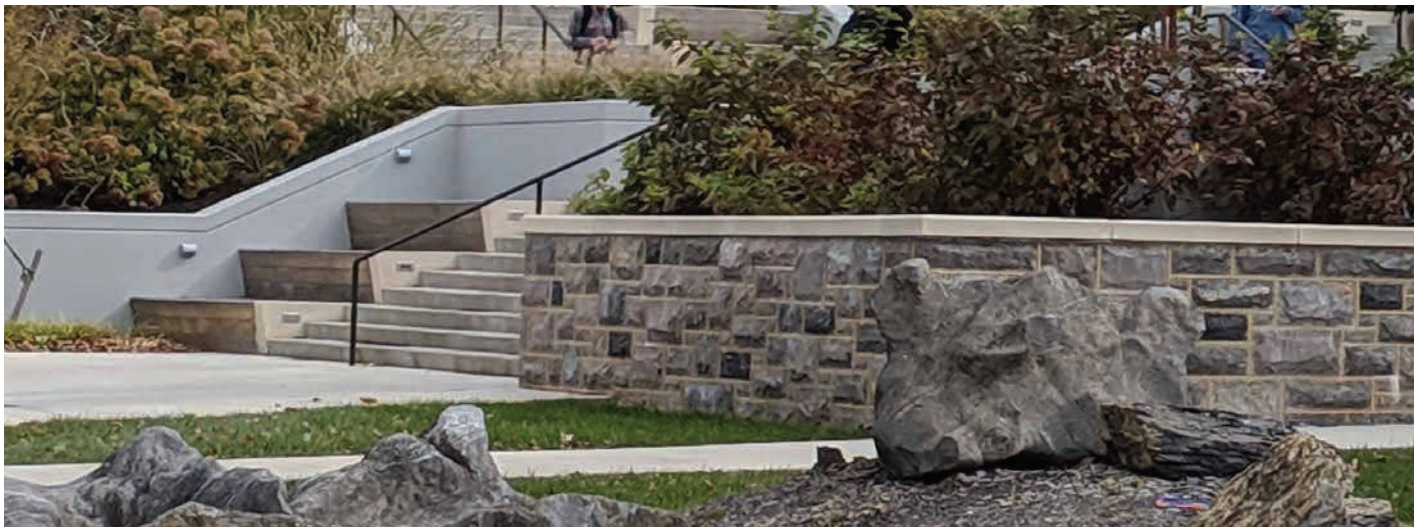
The newly renovated staircase outside Derring Hall improves the appearance, function, and safety of one of the most heavily trafficked areas on campus.
