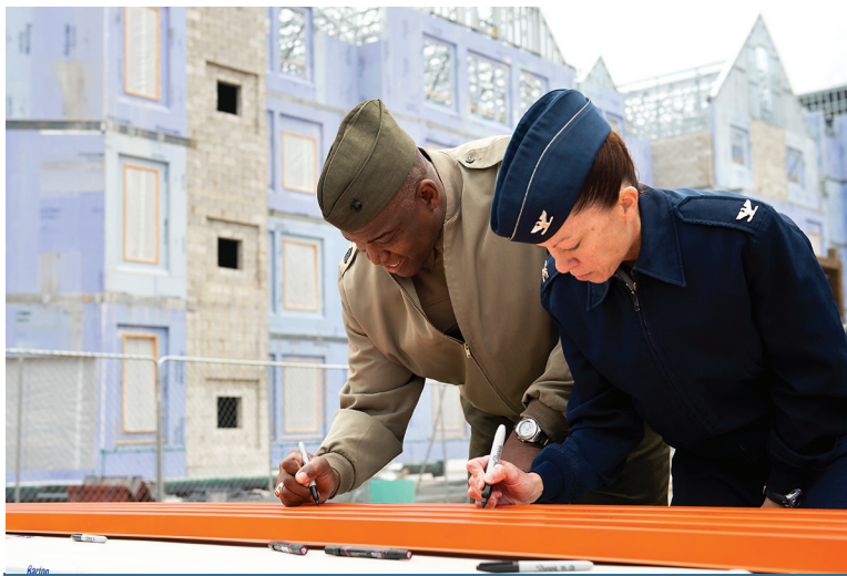
Members of the Virginia Tech Corps of Cadets sign beams that became part of Pearson Hall, the new upper quad residence hall built in fiscal year 2016.
