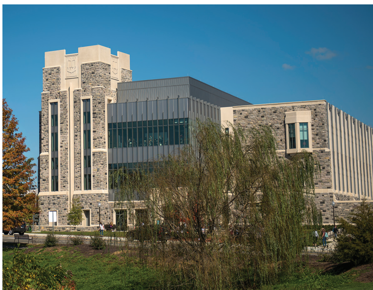
The new classroom building constructed during fiscal year 2016 incorporated a traditional Hokie Stone exterior with modern design to support interactive learning experiences and meet LEED standards.
